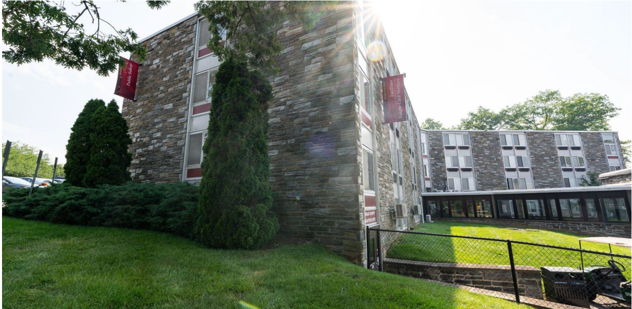
Dilworth Hall, Public Safety Entrance
